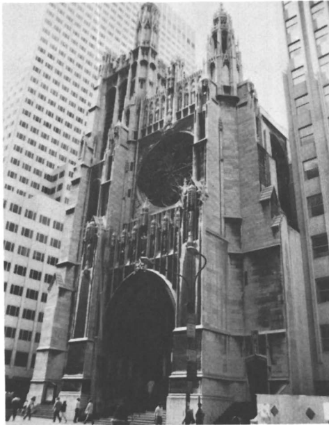
St. Thomas Church in New York City. Areas on the facade accumulate a layer of gypsum (calcium sulfate) produced by acid deposition attack on the limestone and then darken by dirt, soot, and other combustion products. (Photo by Elena Charola.)
